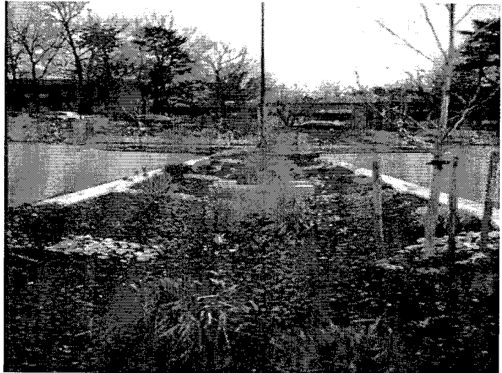
This parking lot island has been designed as a bioretention facility. Runoff is directed into the shallow landscaped areas where treatment is provided.
