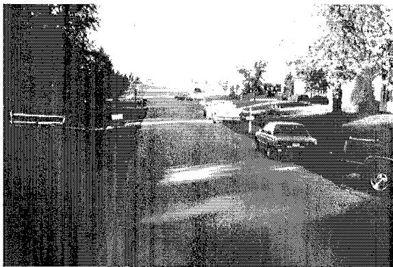
Narrow residential streets reduce traffic speeds, improve safety, provide sufficient access and parking, and reduce the amount of impervious cover created.
