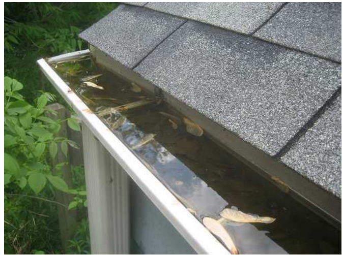
Figure 19. Clogged rain gutter filled with water ( http://www.moonworkshome.com )
