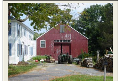
This outbuilding in the Old Town Center Historic District in Winchendon is still used for agricultural purposes.
