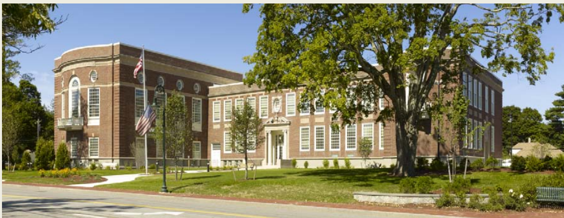
After sitting vacant for 30 years, the Wilbur School in Sharon was proposed for demolition in due to its condition. It has since been rehabilitated into housing and has received an MHC Preservation Award.
