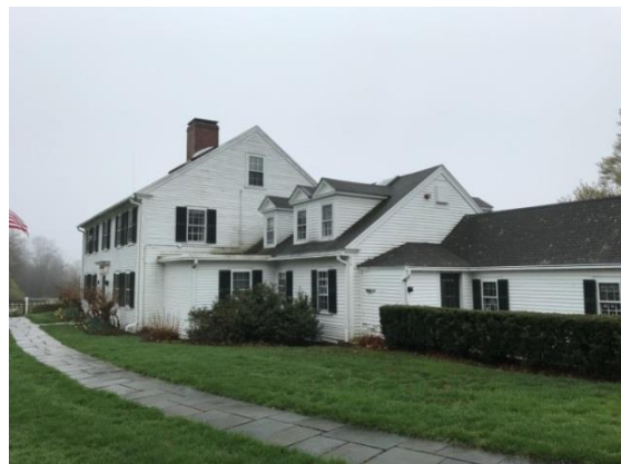
Patton Homestead North Elevation
