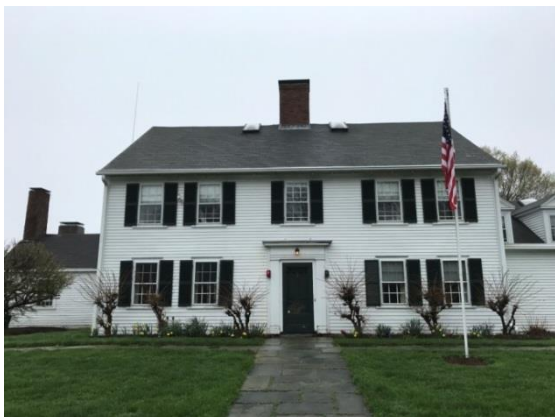
Patton Homestead East Elevation 650 Asbury Street
