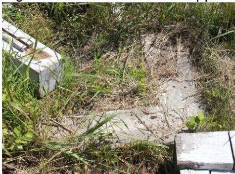
4. Contractor to supply & install all new cedar 6" x 6" vertical support posts (28) which supports the canopy at approximately the same location as the existing supports. Contractor should use fasteners to secure the new posts to the concrete foundations.
