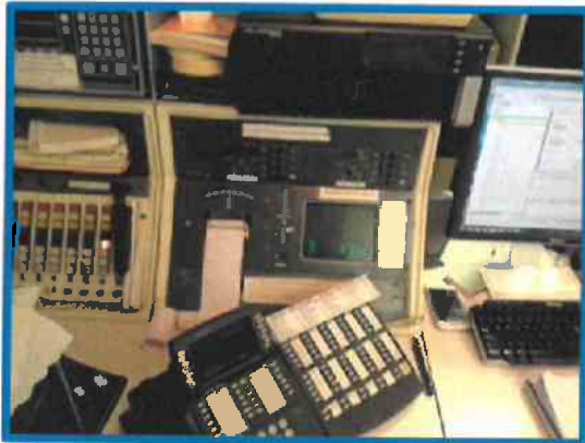
Figure 22: Keltron fire alarm panel in Danvers dispatch center.
