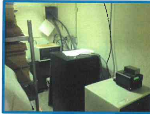
Figure 5 (left): Transmitting phone lines in basement of Danvers PD connecting radios to various remote sites. Limited coverage from this site due to height of tower.
