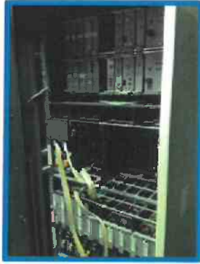
Figure 5 (left): Transmitting phone lines in basement of Danvers PD connecting radios to various remote sites. Limited coverage from this site due to height of tower.
