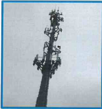
Figure 3 (left): 130' cell tower at former Danvers State Hospital site with police and fire antennas mounted on it. Figure 4 (right): UPS battery back-up power units at former Danvers Hospital site which provide redundancy in the event emergency generator also fails during a power outage. Fire and police radios each have a UPS unit which can provide up to 12 hours of power.
