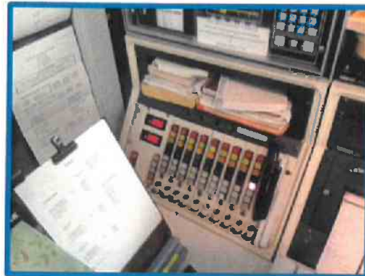
Figure 23: L.W. Bills fire alarm master panel located in Danvers dispatch center.
