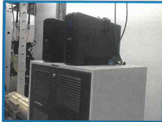
Figure 3 (left): 130' cell tower at former Danvers State Hospital site with police and fire antennas mounted on it. Figure 4 (right): UPS battery back-up power units at former Danvers Hospital site which provide redundancy in the event emergency generator also fails during a power outage. Fire and police radios each have a UPS unit which can provide up to 12 hours of power.
