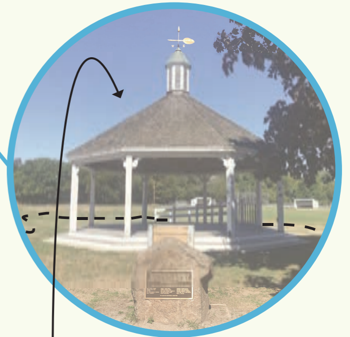
Main gathering space is undefined and gazebo is in need of repairs.
