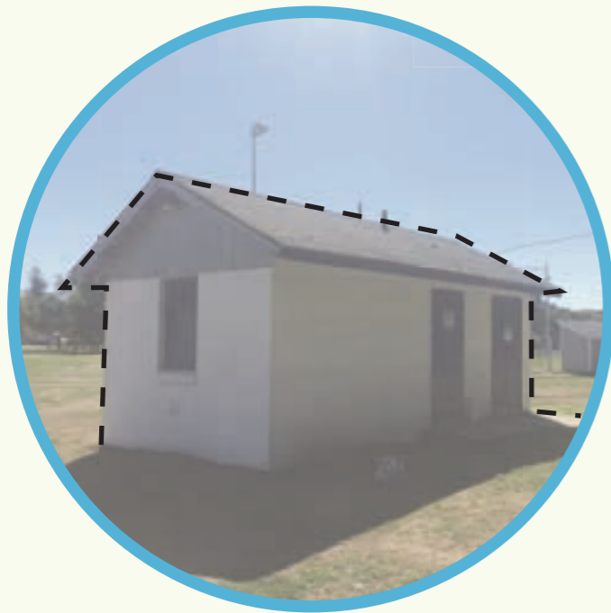
Bathroom building is outdated and in a location disconnected from highly used park spaces like the playground.
