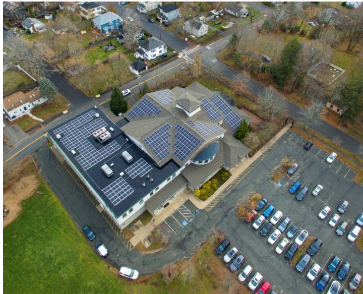
Rooftop Solar PV Array on Roof of HW Library
