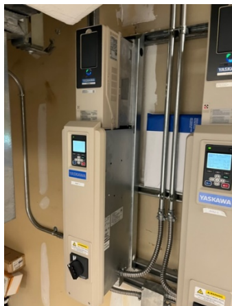
Two new VFDs at PSB for AHU-1
